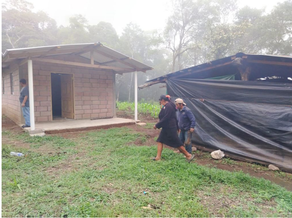
- THE NEW HOUSE NEXT TO THE PLASTIC HOUSE -
