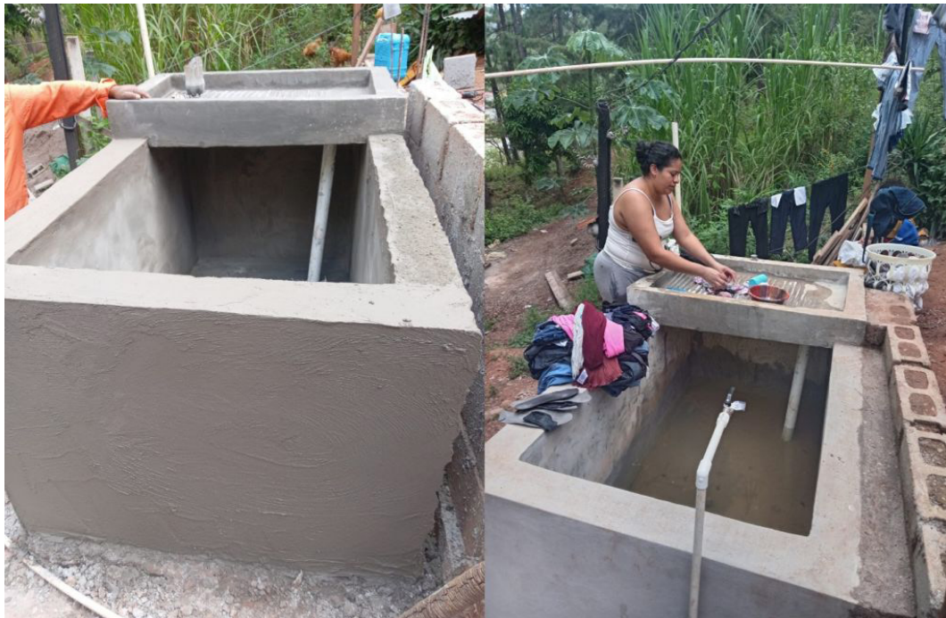
- A COMPLETED PILA -
