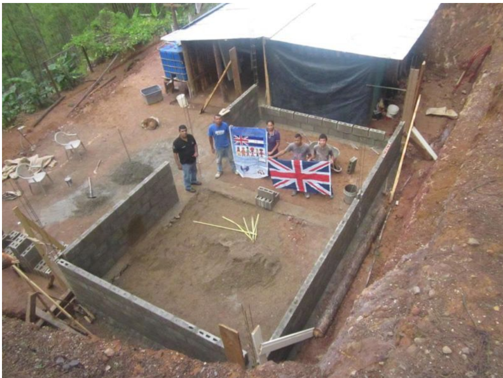
- A NEW HOUSE UNDER CONSTRUCTION WITH THE CURRENT HOUSE MADE OF WOOD AND TARPULINS BEHIND -
