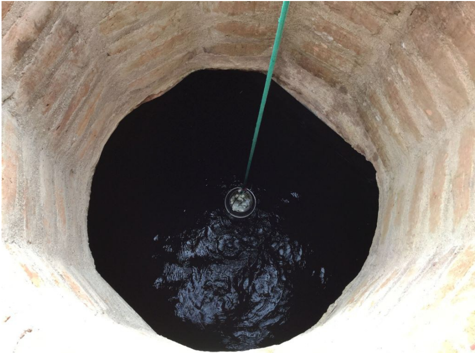
- THE COMPLETED WELL -
