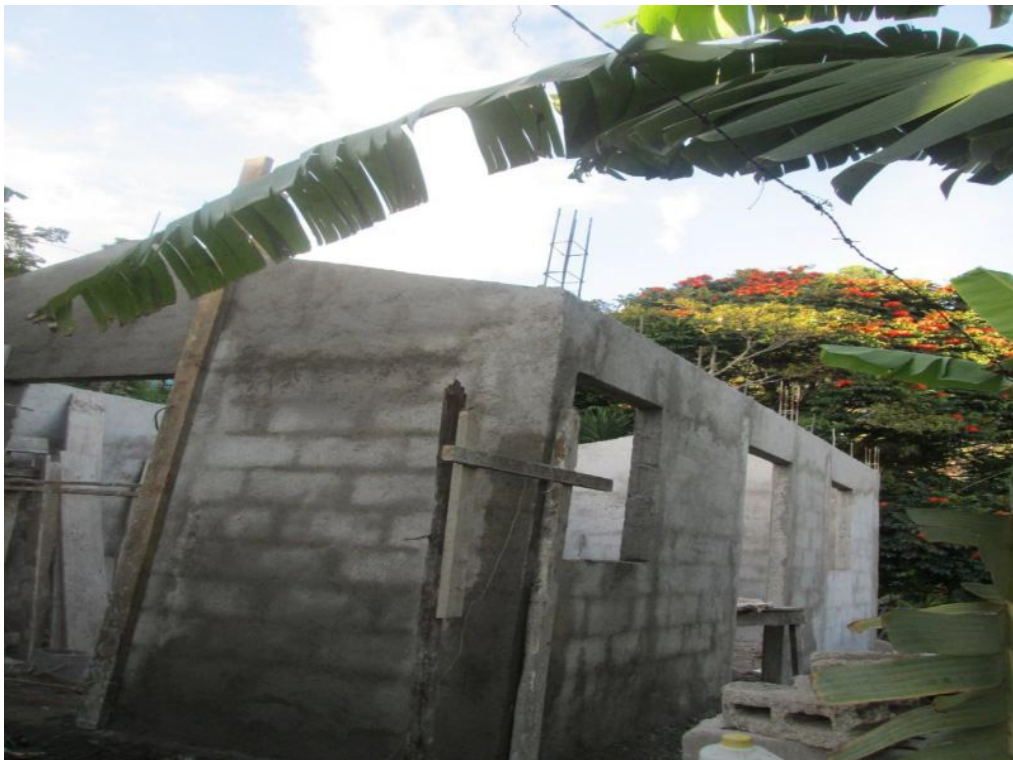
- THE REPLACEMENT HOUSE BEING BUILT -
