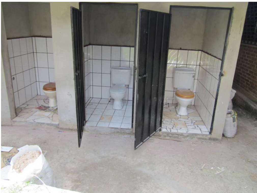
- THE FINISHED TOILET FACILITIES -
