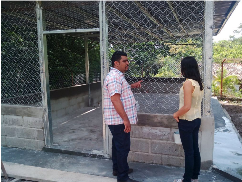
- NEW HEN HOUSE AT GUANACASTE SCHOOL -
