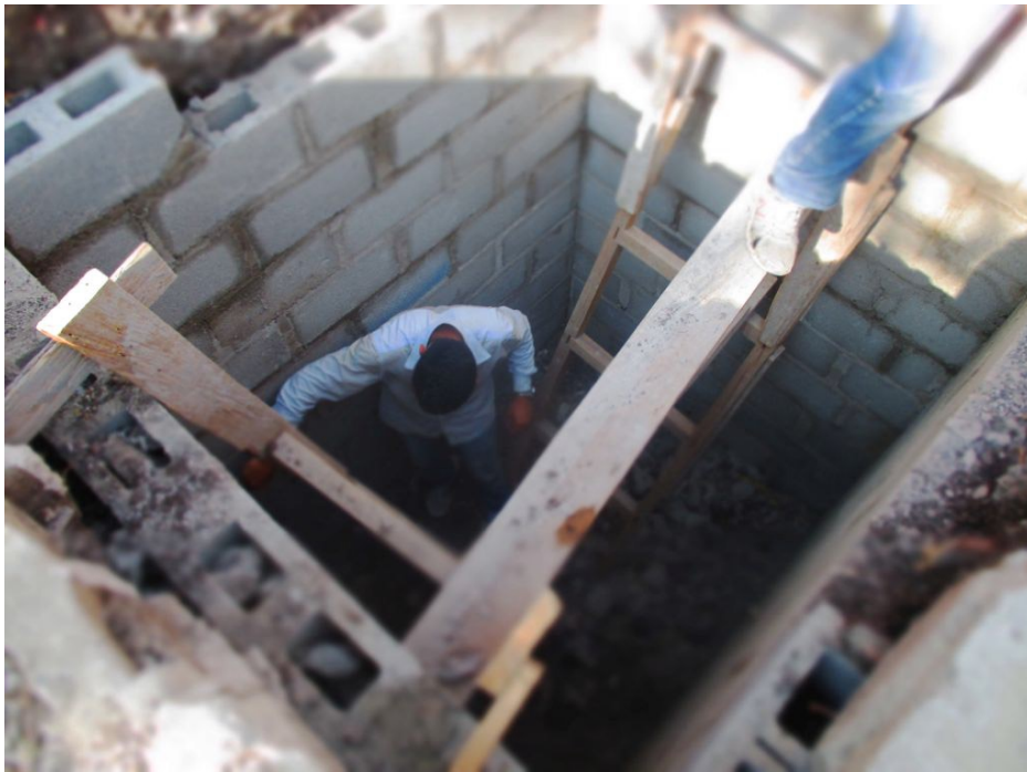
- BUILDING THE SEPTIC TANK AT FUNEZ -
