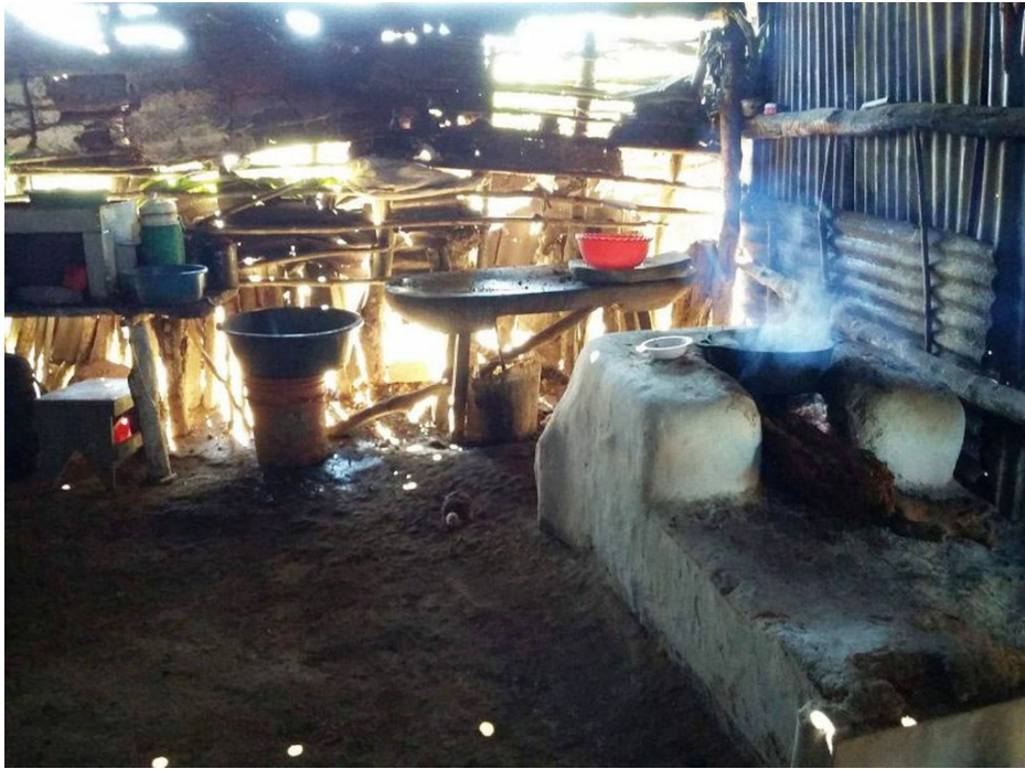
- THIS HOUSE IS OPEN TO THE ELEMENTS -
